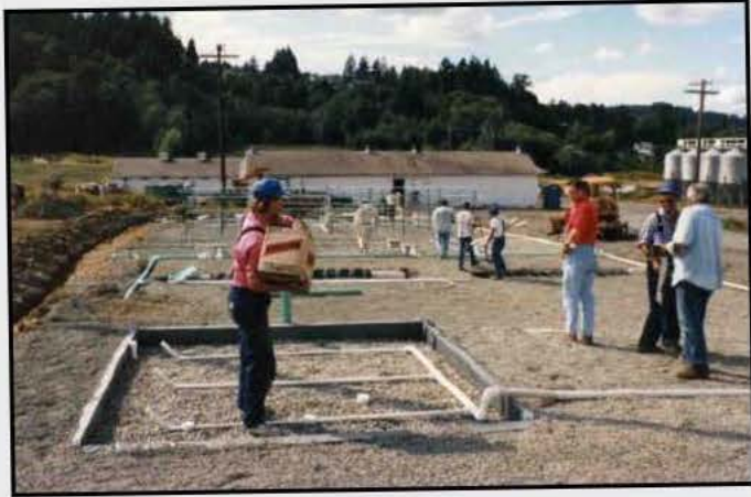
A recirculating gravel filter under construction.
