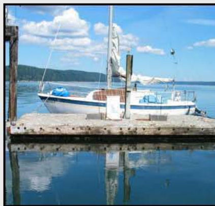
Vessel holding tank pumpout station at Twanoh State Park.
